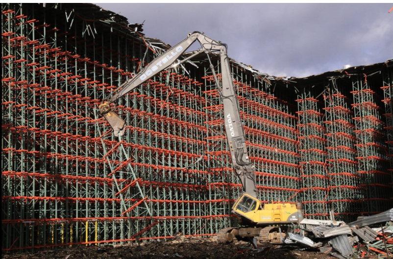
Demolition of the rack system
